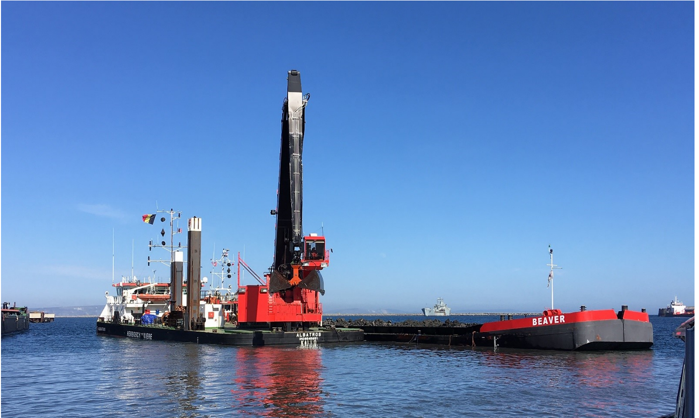
Picture: Dredging being carried out on Outer Coaling Pier (OCP)
